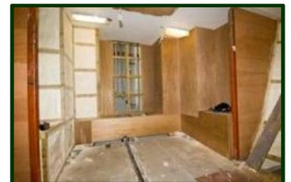
In the second stage, wooden grounds were placed on the sides and bulkheads of the hold which were filled with spray foam to a thickness of up to sixty inches in places where they had to build boxes out so the fish boxes in the hold remained in place once they were stored. Following the application of spray foam the joiners placed plywood on top of the insulation which was coated with a fibreglass gel coat for water proofing purposes.
